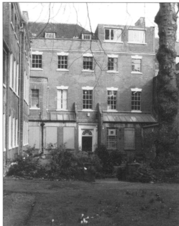
Fig. 2 Rear view of Bromley House. The meridian line is in the room with the shutters partly closed: the aperture will have been in the upper part of this window.
